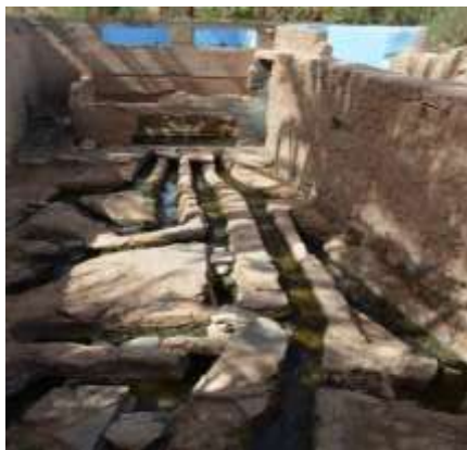
Figure 26: Hydraulic networks connected to the collection basin for watering the orchards, Ikoudass – Tzadart.
